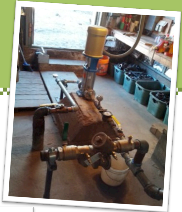
NEW TRANSFER PUMP INSTALLED.
