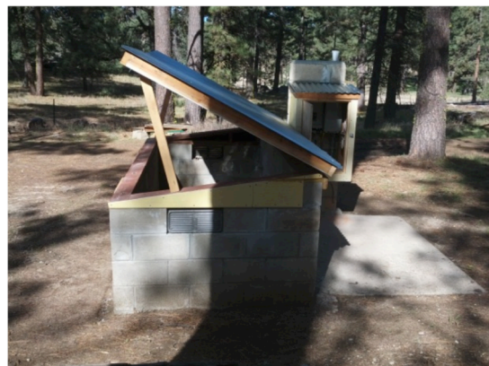
New wellhead housing recently completed.
