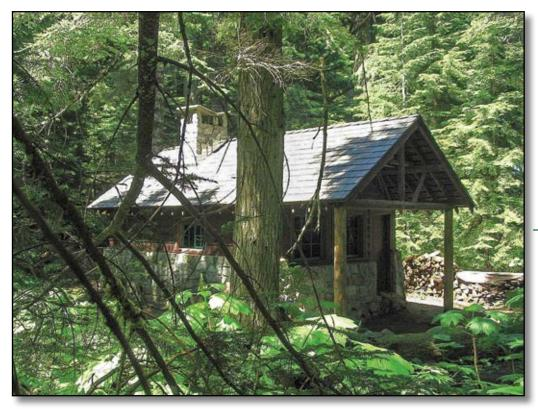
Figure 8—A tree fell during a storm and destroyed most of the original roof of this 1950 recreation residence at the Denny Creek tract of the Mt. Baker-Snoqualmie National Forest in the Pacific Northwest Region. The new roof structure and materials match the appearance of the historic roof, although the structure was strengthened to meet code requirements for snow loading.
