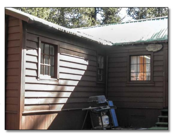
Figure 5—Part of the windowsill broke off of this recreation residence's left window. Replacing it with a windowsill that exactly matches the other windows is routine maintenance. • Similar activities that don't visibly change the exterior of the building or include structural changes
