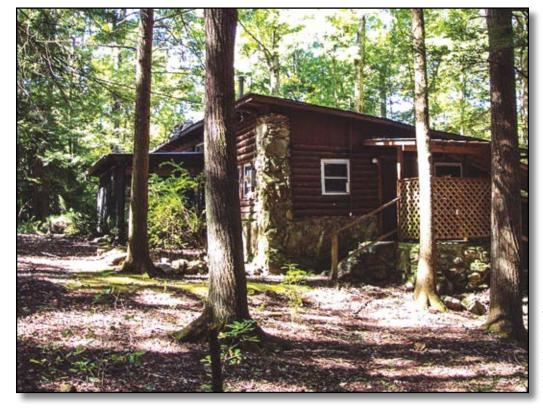
Figure 14—Natural stone was used at the corners, on the lower portion of the walls, and as the foundation for this recreation residence at the Pisgah National Forest in the Southern Region.
