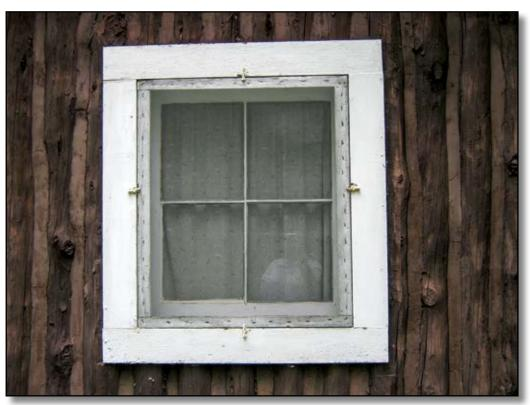
Figure 15—The screen on this small divided-lite window keeps bugs out when the window is open during the summer. The screen is attached using four pivoting double wing screen clips for easy removal. The 1958 recreation residence is at the Rollways tract of the Huron-Manistee National Forest in the Eastern Region.
