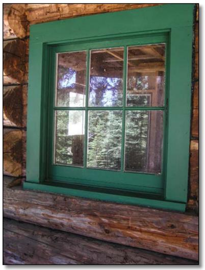
Figure 6—This window on a cabin at Adams Camp of the Nez Perce National Forest in the Northern Region was rebuilt to match the historic window, installed in the original window opening, and painted the original color. Window replacements that match the historic windows are minor changes.
