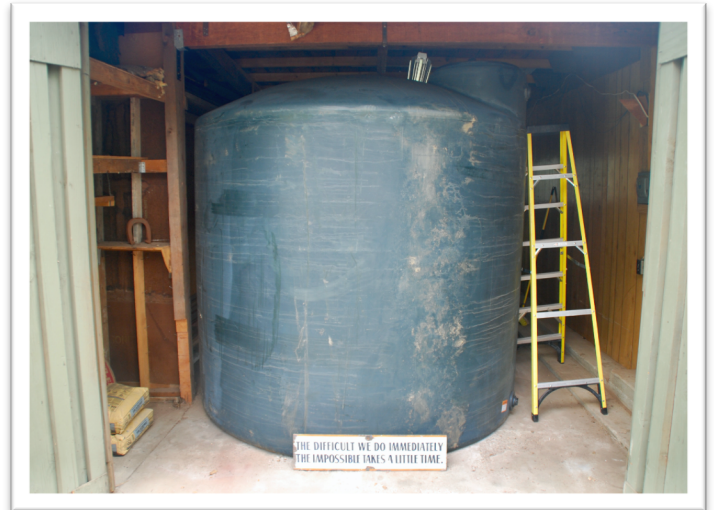
Current water holding tank for Shrine Tract cabins.
